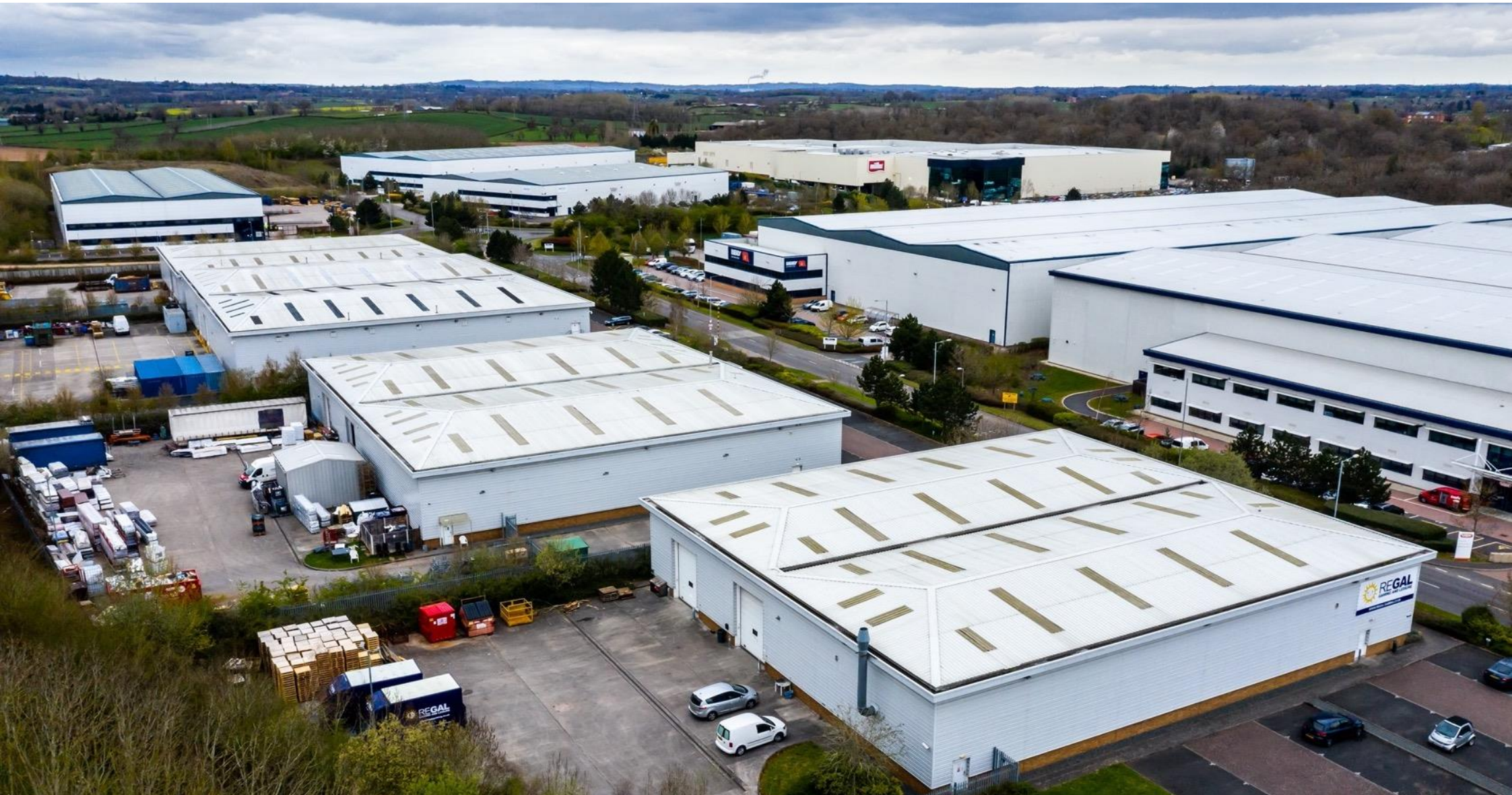
Stonebridge Cross Business Park, Droitwich Spa
